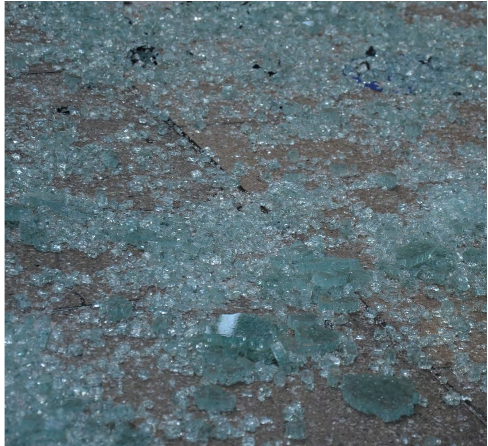
Figure 6: Glass fragments from broken glazing panel strewn over the floor following the panel failure. Large chunk fragments can be seen mixed with smaller fragments.
