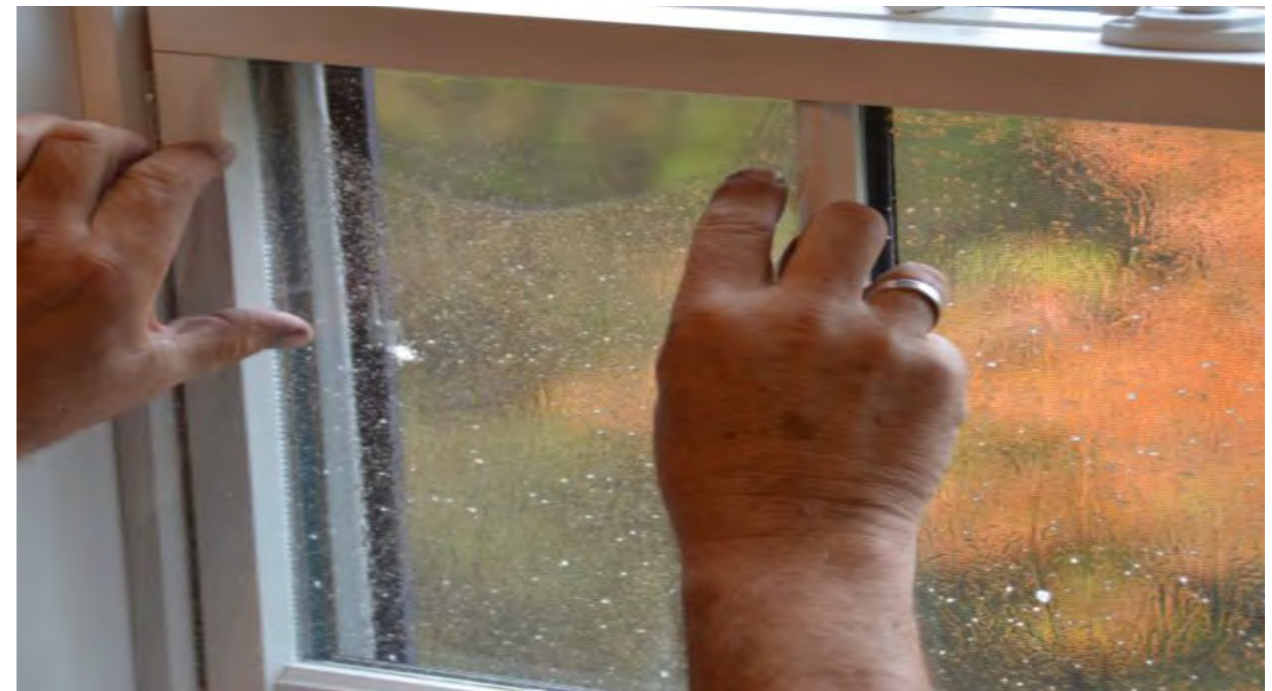
Figure 21: Alternative wall glazing solution examples: (top) architectural mesh. (bottom) safety film being applied to glazing
