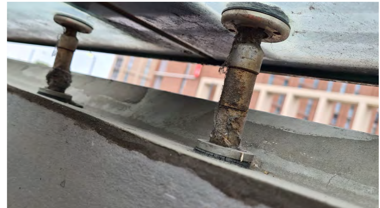
Figure 24: The canopy roof glazing is open, allowing unrestricted air circulation within the Bus Station.
