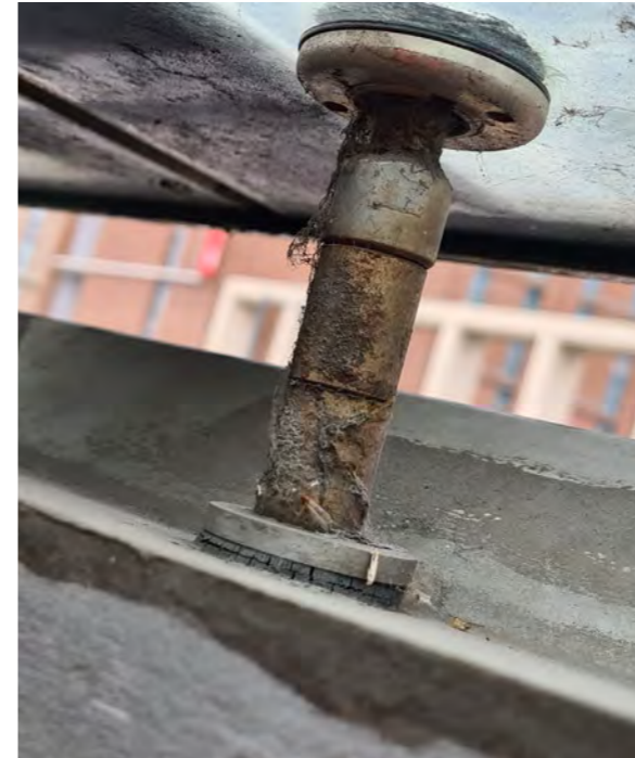
Figures 9-10: Left: Spider fitting viewed from underside of glass panel, showing pronounced corrosion on spacers, severely degraded bush between fitting and steelwork, and dirt accumulation. Right: Spider fitting from failed glass panel. Ball-joint appeared seized as it couldn't be moved by hand.
