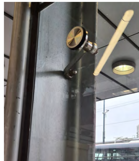
Figures 19-20: Left: Top spider fitting on vertical glazing panel. Right: Vertical glazing walls are composed of two glass panels on top of each other.
