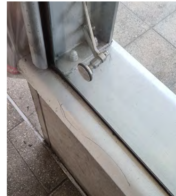
Figures 17-18: Left: Vertical glazing corner to waiting area of Station. Right: Spider fitting on vertical glazing. Both photographs show the plinth offsetting the glass panels from the ground floor.
