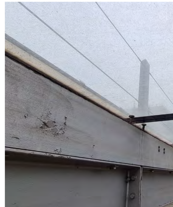
Figures 11-12: Left: Steelwork structure showing flaky coating. Right: Spider fitting on lower edge of glass panel, also showing a severely failed bush, and general dirt accumulation.
