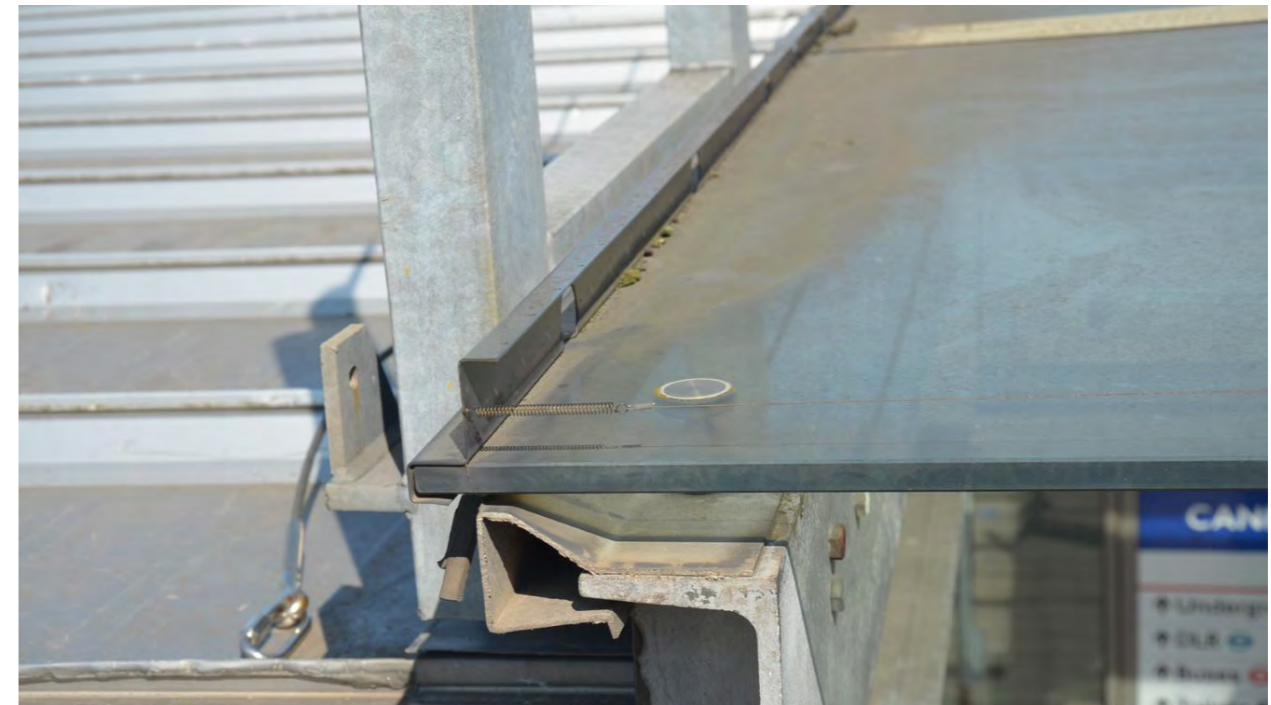
Figure 7: Overhead glazing panel in place. Also visible are the fixing system, glazing bar, and tensioning wire.
